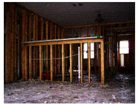
Moldy walls removed, MS
